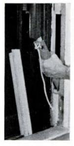
6 Lift counterweight from its box as the first step in replacement of cord. To reach weight, you must pry out box lid, shown at left. Screws sometimes hold in the lid.
