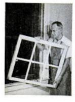
4 Upper sash then comes free. As first step in curing binding, or preventing it, sand the vertical edges of both sashes and the frame channels in which they run. Give extra attention to rubbed spots, a sign of binding.
