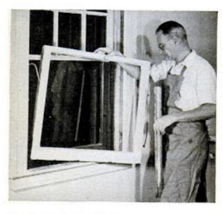
2 Lift out the lower sash after bead and remaining cord have been removed. If there's a metal weather strip, take this out too. Small nails hold it down.
