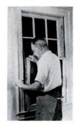
10 Repeat process for the bottom sash after tacking back the parting strips. Be sure to fasten the chain with a screw, for driving in a nail might crack the glass.
