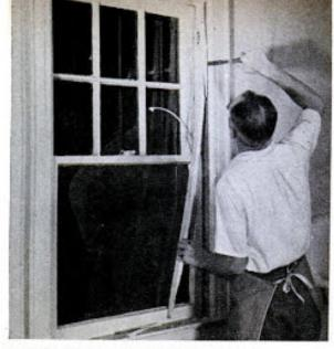
1 Pry off stop bead that retains lower sash. It may split, but you can replace it inexpensively. If one cord is still good, mark it so you can replace in same position. Loop end to keep it from dropping inside weight box.
